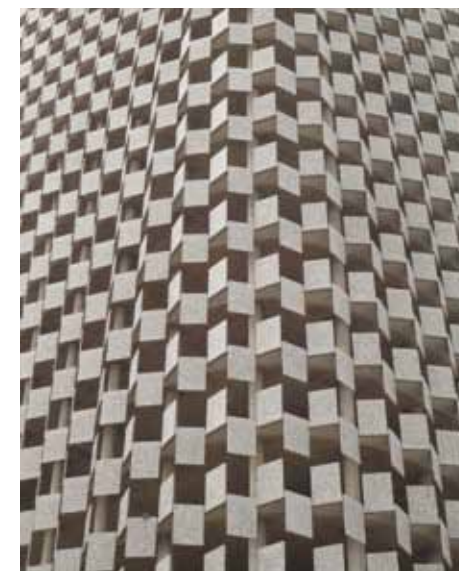
A skyscraper under construction – JvM
