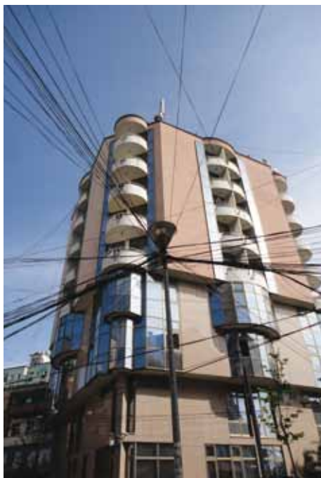
Creative wiring solutions - JvM
